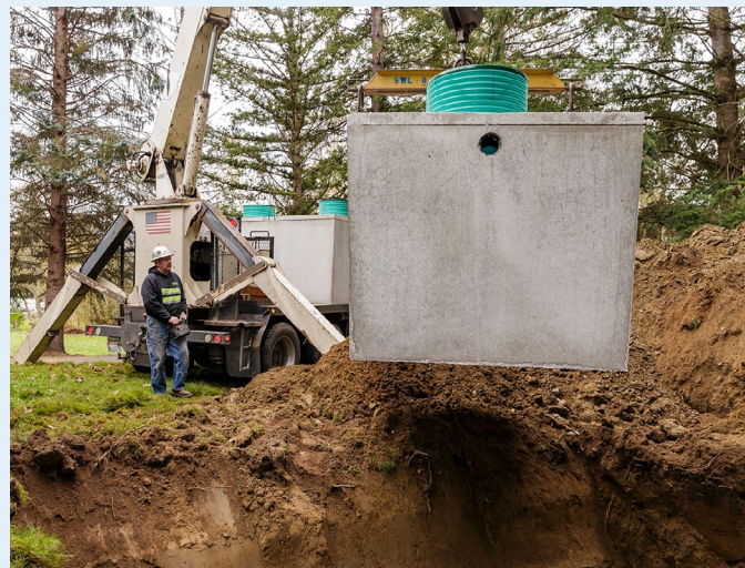
Septic replacement in Washington state.
